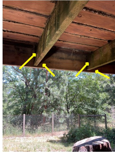
Back deck is missing proper brackets where floor joist attached to rim joist, starting to twist, recommend update by licensed contractor.
