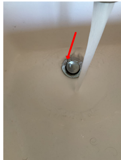
Upstairs master bath left sink has a cracked drain coupler, appears to be no active leaks where visible, repair/replace as needed.
