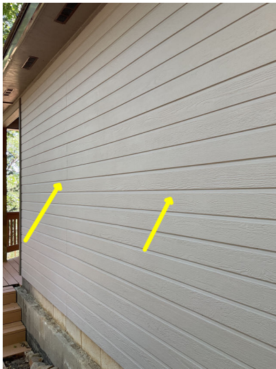
Most Siding has general minor wear/moisture damage from age, recommend monitor, prep/paint as needed.
