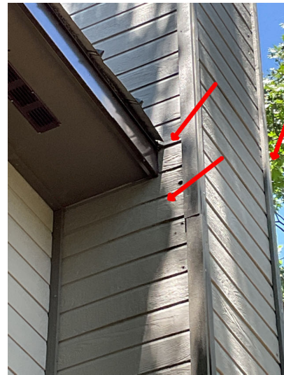
Right, Moisture damage siding starting around chimney at roof level, no kick back flashing or gutters in place. Recommend install.
