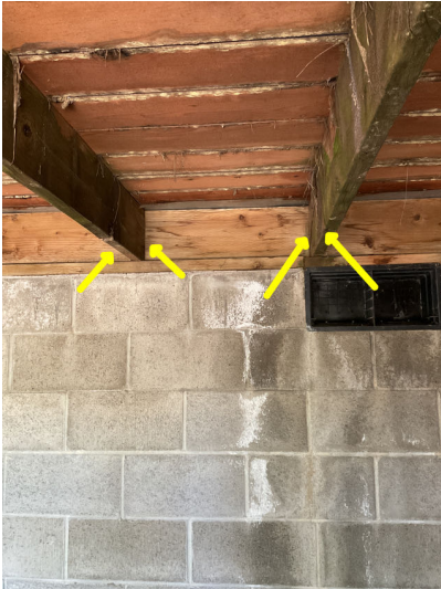
Back deck, improper ledger board and missing proper brackets where floor joist meet ledger board, recommend install by licensed contractor.
