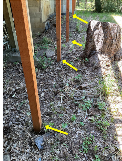
Back deck has wood to soil contact, appears to have concrete footings, recommend clean soil away for proper air gaps .
