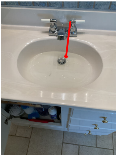
Upstairs bath three has a slow drain at sink, recommend repairs by licensed plumber.
