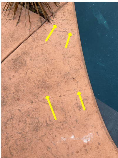
Minor common settlement cracks noted, recommend monitor over time for any further expansion.
