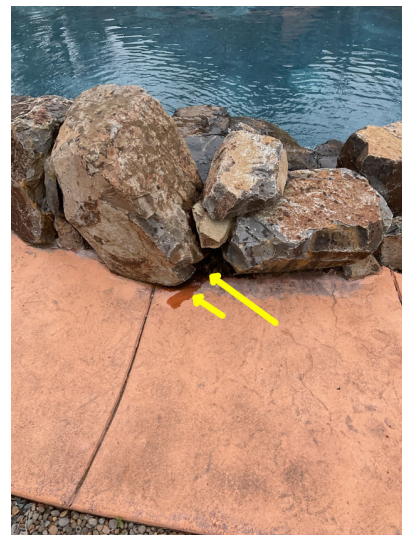
Large Water fall is functional but appears to have a minor leak at back of rocks onto paving/pool deck,
