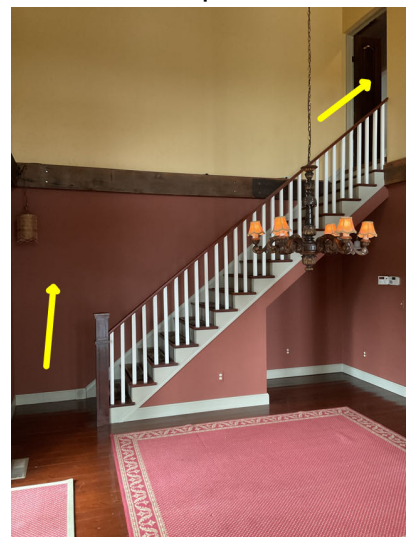
No three way light switch at top/bottom of stairs, update if wanting to meet today's safety standards.
