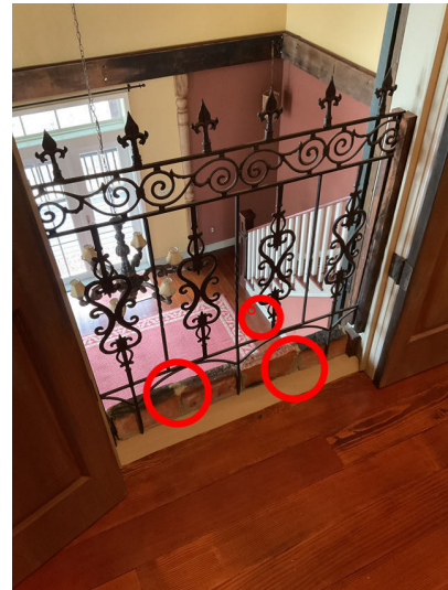
Upstairs hall opening has loose hand rail/spindles, & gaps that exceed 4 inches, recommend update, especially if small children will be present.
