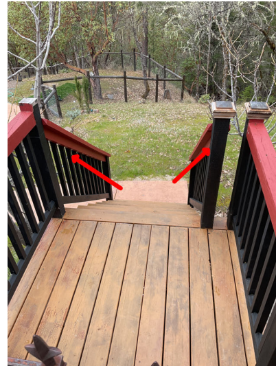
Both Exterior back stairs hand rail is starting to get loose, recommend re secure for safety by licensed contractor.
