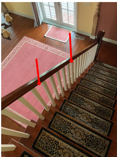
Interior stair hand rail starting to get a little loose, recommend re secure or have assistance by licensed contractor.
