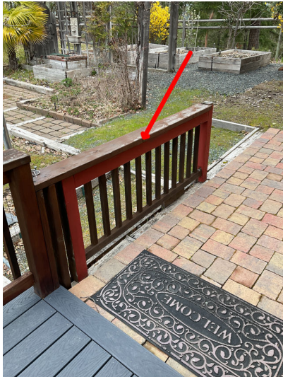
Exterior right, small section of hand railing loose, recommend re secure or contact licensed contractor for repairs.
