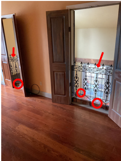
Upstairs left bedroom has cut outs, openings with hand rail that's loose, & gaps exceed 4 inches, this is a potential safety hazard.
